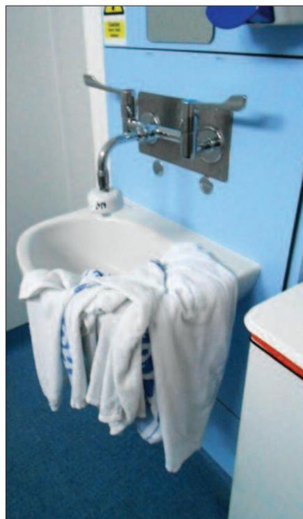
*A handwash basin used inappropriately for storage of used towels. Note the point-of-use filter fitted to prevent the release of *Pseudomonas aeruginosa* due to repeated colonisation of the outlet.*
